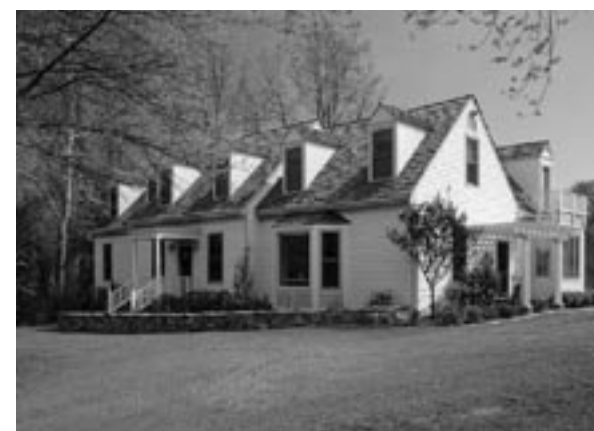
Waiver House Middleburg, Virginia
