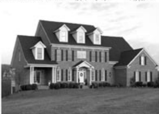
WATERFORD HEIGHTS - Custom built, all brick 4 level, sun-filled home on almost 4 acres with mountain views. 6 bedrooms each with its own bath. 2 story foyer & great room open to stunning kitchen with cherry cabinets and black granite counters. Hardwood floors, 3 fireplaces, sunroom and study on main level. Porches, decks and balcony bring the outside in. $2,200,000. Please call Michele or Andy Stevens at (540) 592-9544
