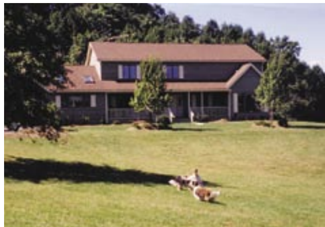
Dixons Mill Marshall, Virginia
