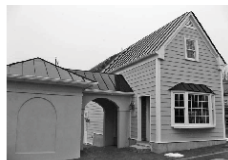
Commercial Building Middleburg, Virginia
