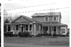
Seaton Store Rectorville, Virginia
