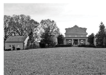
Manor House at Chattin's Run Delaplane, Virginia
