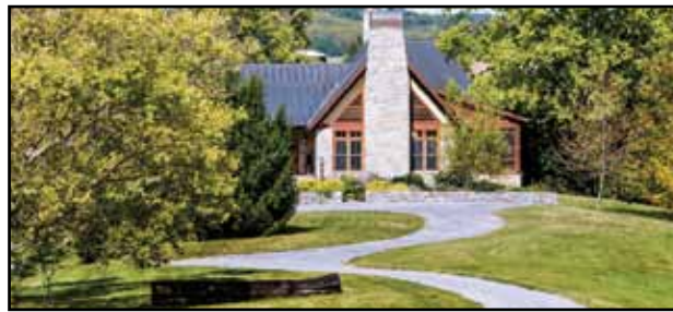
2909 MILLWOOD ROAD – MILLWOOD – SOUTH GATE FARM. A BEAUTIFUL TURKEY HORSE FARM, IS LOCATED ON THE EDGE OF THE CHARMING VILLAGE OF MILLWOOD. THIS UNIQUE PROPERTY CONSISTS OF 126 ACRES OF PRIME LAND IN CONSERVATION EASEMENT DESIGNED TO CATER TO THE HORSE AND THE HORSEMAN. A CUSTOM STONE AND STUCCO HOME BUILT IN 1999 WITH NO DETAIL LEFT UNTURNED -- 4,300 SQUARE FEET INCLUDING A GOURMET KITCHEN, CUSTOM MILLWORK THROUGHOUT, GEOTHERMAL HEATING. CL7939070
