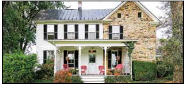
20596 AIRMONT ROAD – BLUEMONT - CLASSIC FIELDSTONE FARMHOUSE ON 5 OPEN ACRES WITH 7 STALL BARN, FULL SIZE DRESSAGE ARENA, VIEWS AND ADJACENT TO MUCH OPEN SPACE FOR RIDE OUT. BEAUTIFULLY LANDSCAPED GARDENS, PRISTINELY MAINTAINED. HOUSE IS AUTHENTIC AND ORIGINAL WITH 4 STUNNING, PLACES. A TIN ROOF, COMPLETELY RENOVATED OVER THE PAST 10 YEARS, WATER AND ELECTRIC TO BARN W/ BOX STALLS, FENCING, PIEDMONT HUNT. LO7928777
