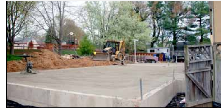
MIDDLEBURG LIBRARY CONSTRUCTION
